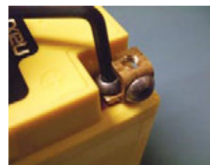
Attaching the terminals
